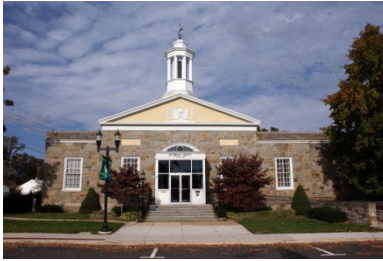
The Historical Society of Harford County, Inc., headquarters.
